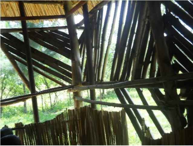
Classroom with a temporary wall.
