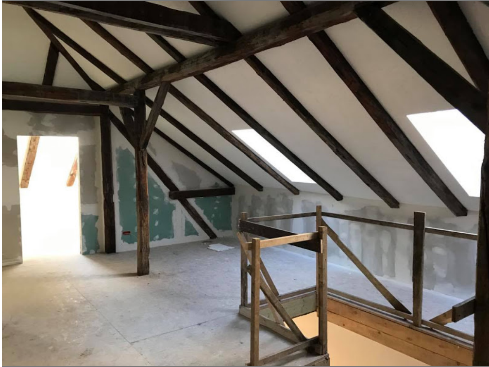
Interior second floor with drywall
