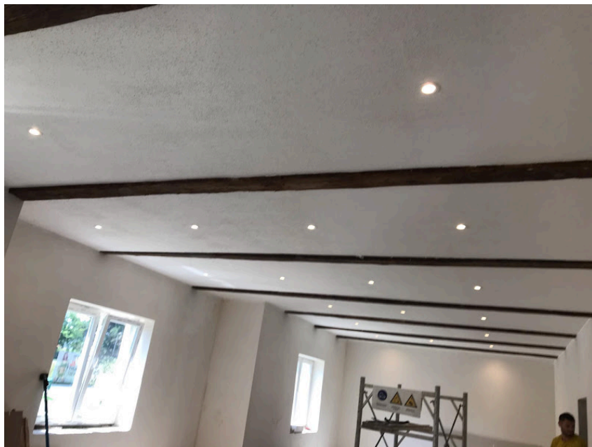
Interior first floor with electrical
