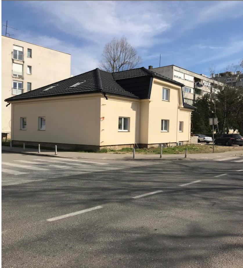
Exterior view from street
