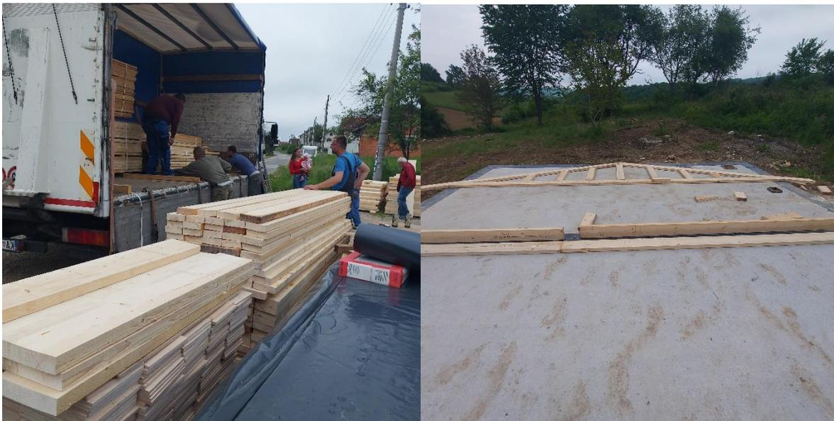
The local workers in Bačuga put the tar down where the walls will go as a barrier between the concrete foundation and the wooden wall frames.
