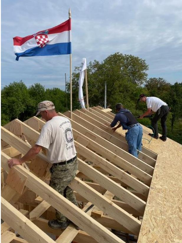
At 16:15 or so a van arrived with OSB . We stacked it up in a good place. He also brought nails for the pneumatic hammer—2 sizes: 5 cm for the roof and tresses and 7 cm for the walls.
