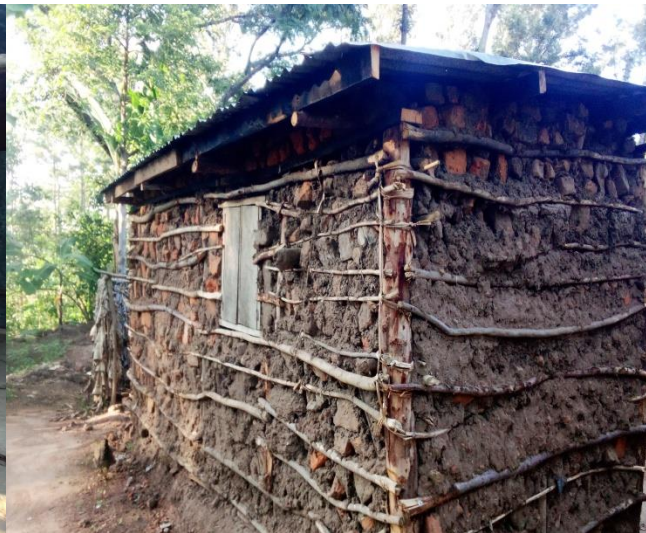
Ms. Aidah's temporally constructed house
