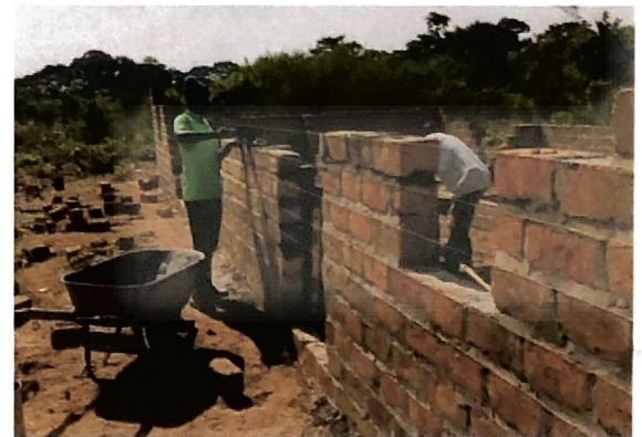
Constructing a home for Pastor Banda
