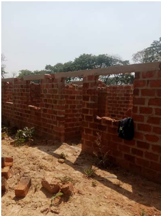
A home in progress
