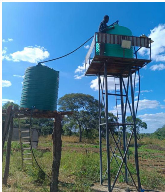
First water tower installed spring 2023
